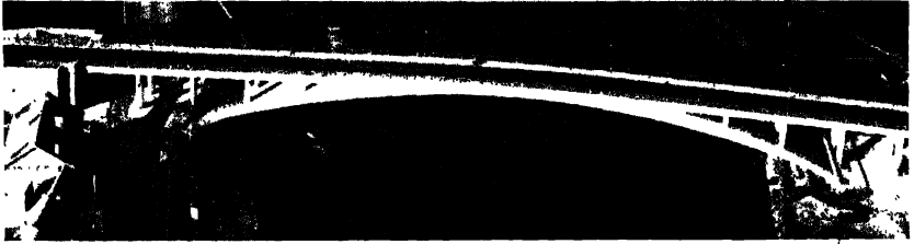
Fig. 365. —Bridge over River Oise at Conflans, France.
